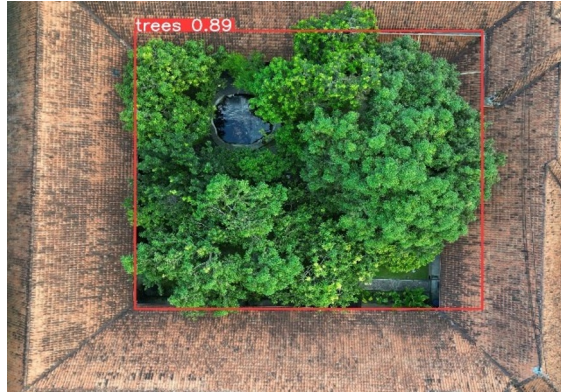
Fig. 5. The tree photo could be separated from the surrounding building.
