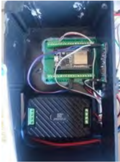
Fig. 3.9. Installation of Box Components 2
