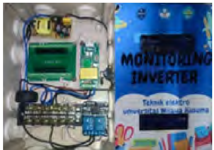
Fig. 3.8. Installation of Box Components 1
