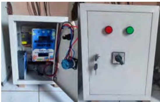
Fig. 3.10. Installation of Mechanical Design
