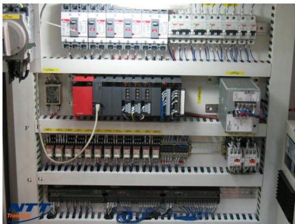
Gambar 12.1. Programmable Logic Controller (PLC)
