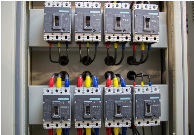
Gambar 4.2. Molded Case Circuit Breaker (MCCB)
