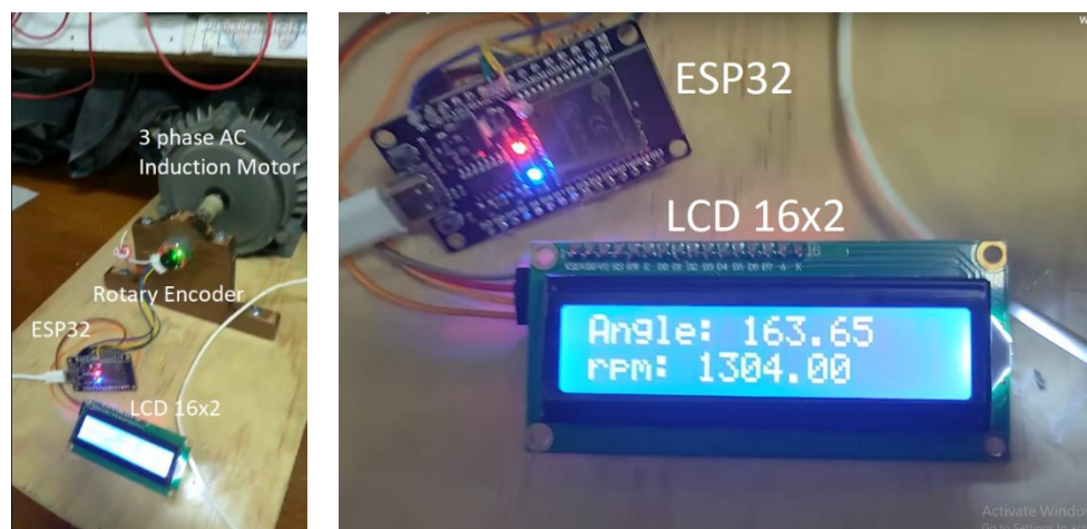
Figure 6. Installation of the rotary encoder on the motor shaft with ESP32 and 16x2 LCD
